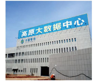
China Mobile data center
